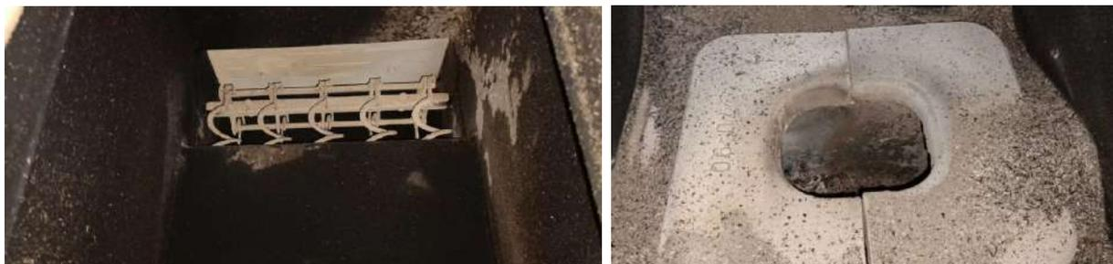
*Figure 6. Images of combustion chamber walls (left) and the lower part of the combustion chamber where the burner is located (right).*
