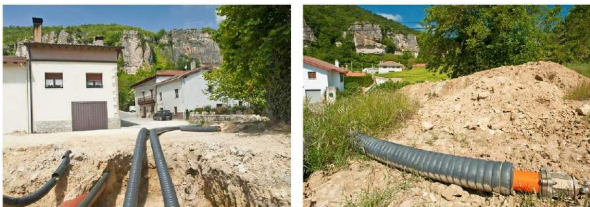
*Figure 52. Civil engineering carried out to develop the district network in Sabando.*
