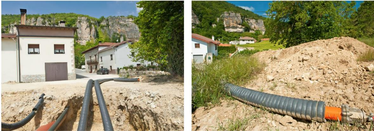
Figure 6. Civil engineering carried out to develop the district network in Sabando.
