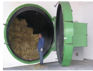
c) biomass boiler
