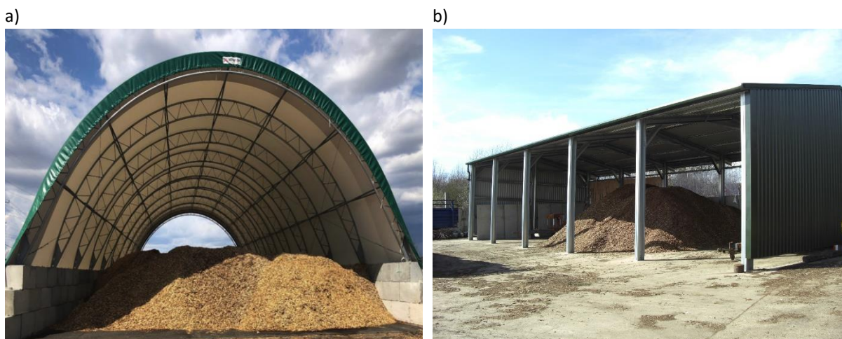
Figure 15. Outdoor chips storages for larger installation [48,49]: a) arched hall; b) shed.
